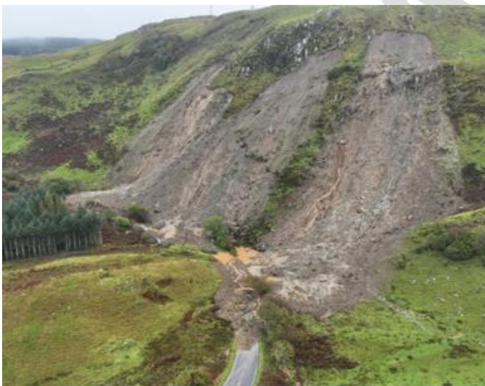
The photo to the left shows the Ardfern landslip on the A816 – c.15000 tonnes of material blocked the road.
